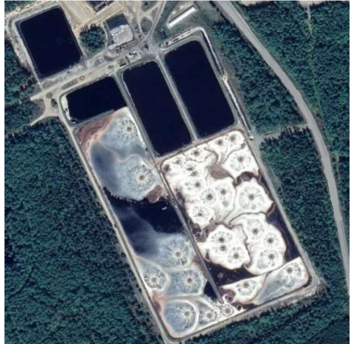
Aerated lagoon installation
